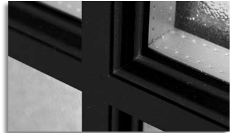
integral spacer bar
